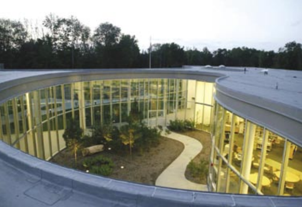
In the exterior courtyards, the curved steel spandrel beams cap the glazed curtainwall system.
